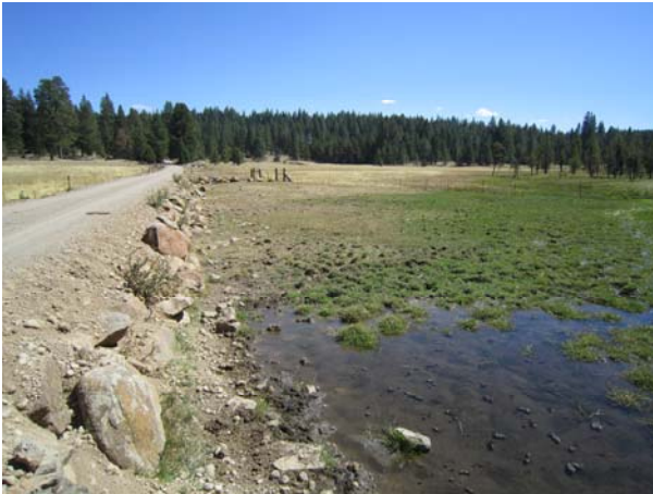
Berms or levees keeping water in wetland
